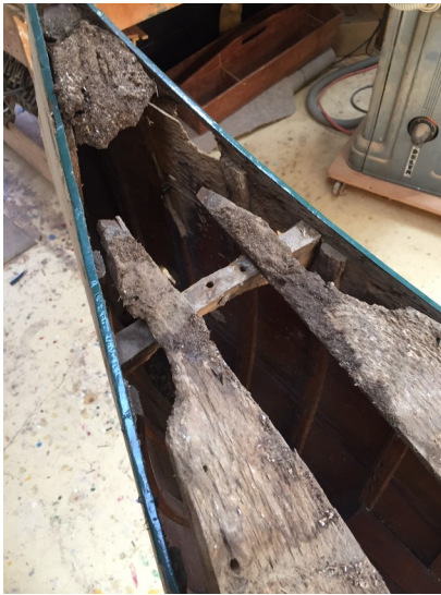
Little remained to show what the decks were like. RC Cross photo
